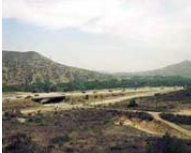
In California's Coal Canyon, a Highway 91 underpass serves as a key connector for mountain lions entering or leaving nearby Chino Hills State Park. Plans are afoot for the state department of transportation to close off the ramp, rip up the asphalt, and turn the underpass into a safe, green thoroughfare not only for the lions but also for various birds, amphibians, and invertebrates.
