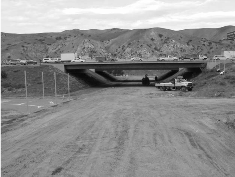
Fig. 22.4. An interchange on the Riverside Freeway (SR 91) being converted into a wildlife crossing in February 2003, to facilitate movement along the linkage between the Santa Ana Mountains and the Chino Hills. Although this is not one of our 15 priority linkages, this illustrates the feasibility of the enhancements that we will recommend in some linkage areas. California State Parks is investing $1.5 million to restore natural vegetation and the Coal Canyon stream channel through the underpass.
