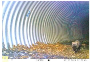
A Pacific fisher passes through an oversized culvert constructed specifically for wildlife west of Redding on State Route 299.
