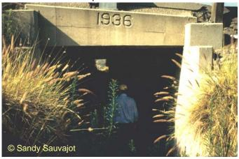
Figure 66. Large concrete box culvert at Conejo Grade.
