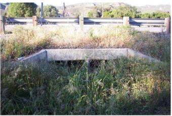
Figure 77. An example of a drainage culvert on State Route 126.
