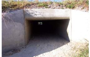
Figure 80. Example of concrete drainage culverts.
