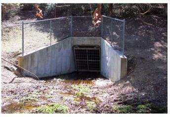
Figure 65. Concrete culvert with trash guard draining Crummer Canyon.
