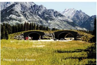
Figure 56. An example of a vegetated land bridge built to enhance movement of wildlife populations.
