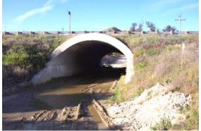
Figure 79. 2-lane arched culvert at Camulos Ranch.
