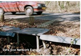
Figure 59. Pipe culvert designed to accommodate small mammals.
