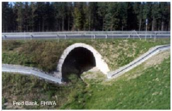
Figure 58. Culvert on German highway, with rail for amphibians and fence for larger animals.
